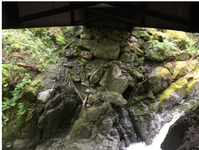
Right Bank Abutment when facing downstream
