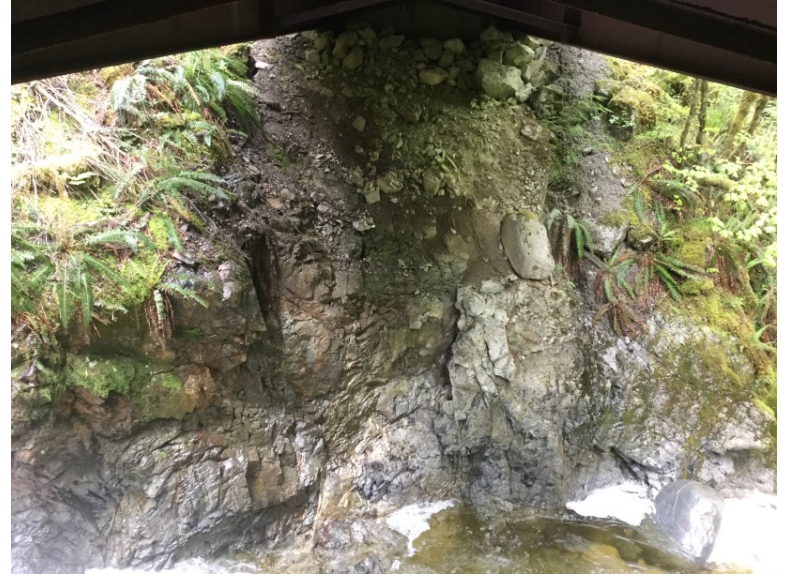
Left Bank Abutment when facing downstream
